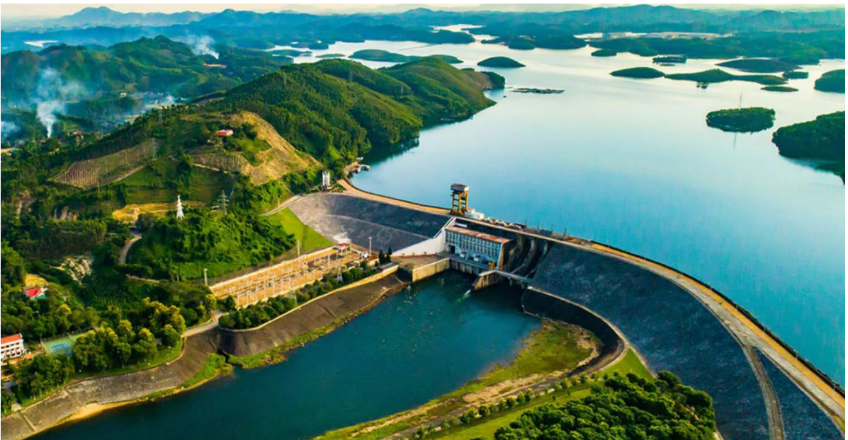
Source: Thac Ba Hydropower Plant 2014, Ree Corporation
